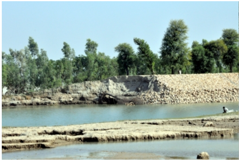
Breached LMB at Taunsa Barrage. (5---11---2010)
