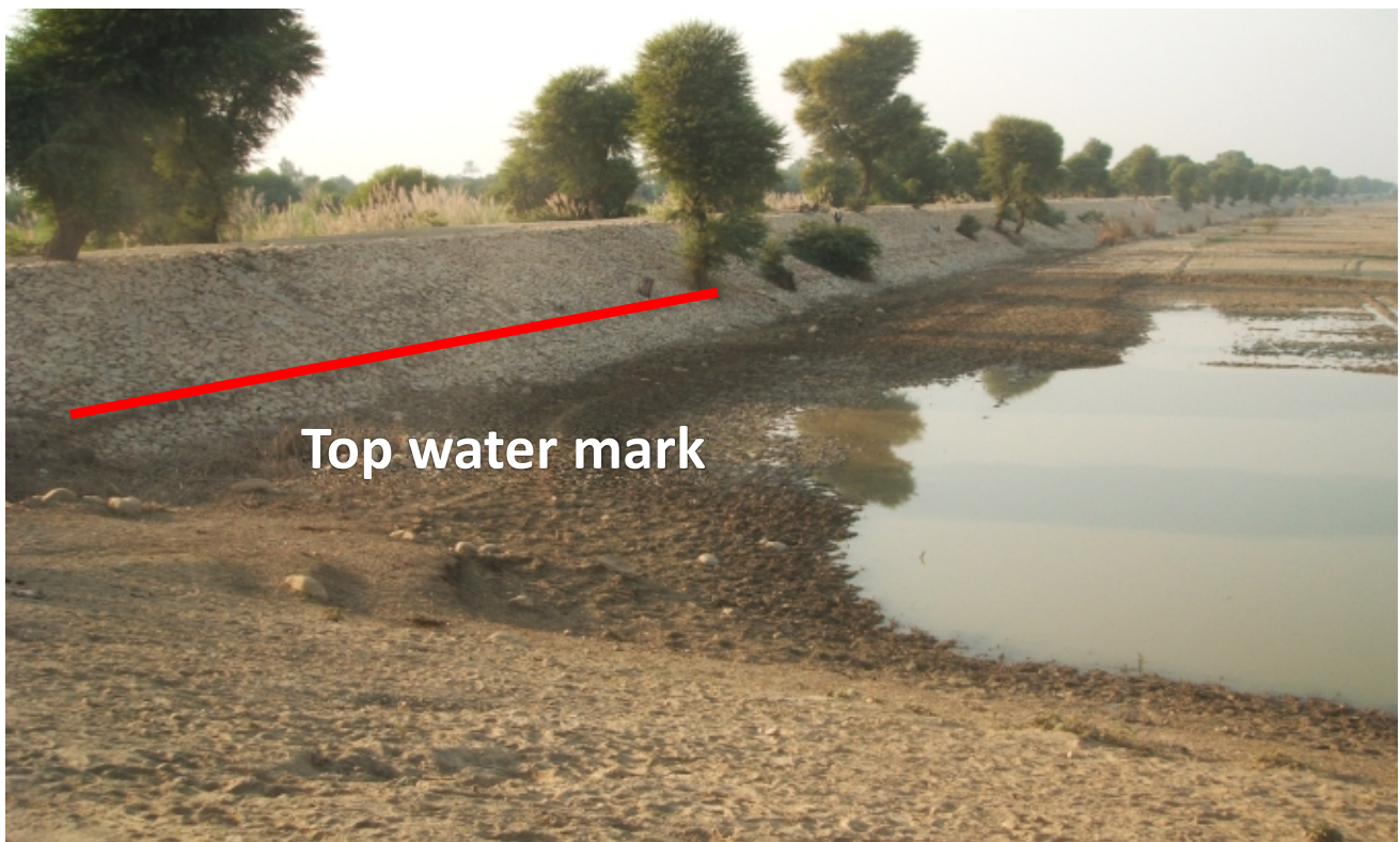
Photo showing presence of flood water in area between Spur # 2-A and Shank of Spur # 2 and water mark on the bank
