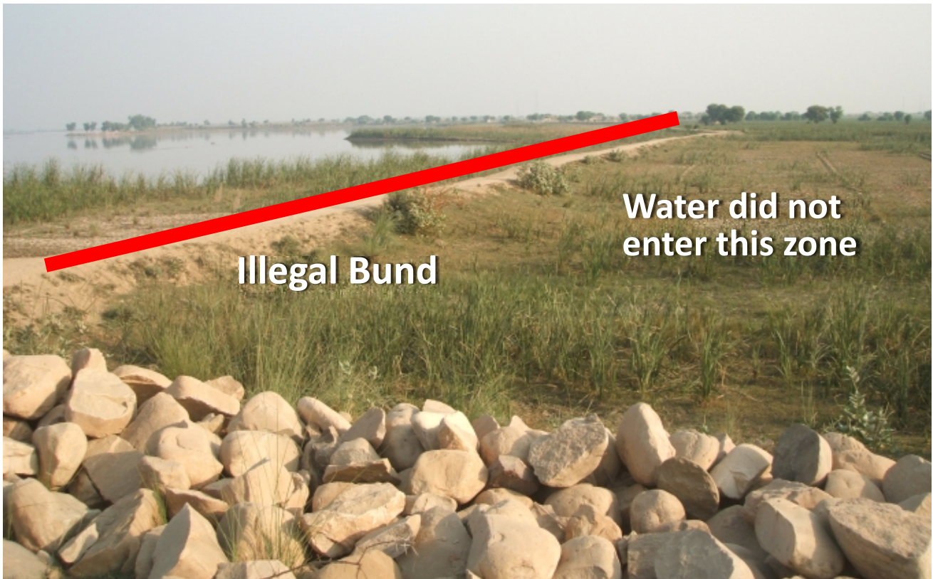
Photo showing presence of illegal bund between Spur # 1-A and T head Spur-5
